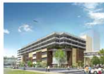
Nagareyama Otakanomori Shopping Center ANNEX
