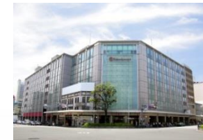
Kyoto Store to be revamped (2023)
