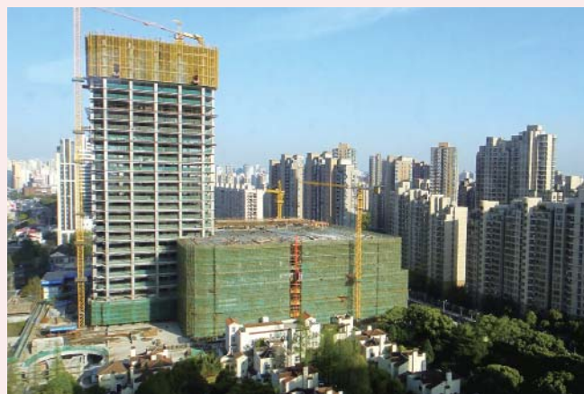
Takashimaya's Shanghai Store, now under construction
